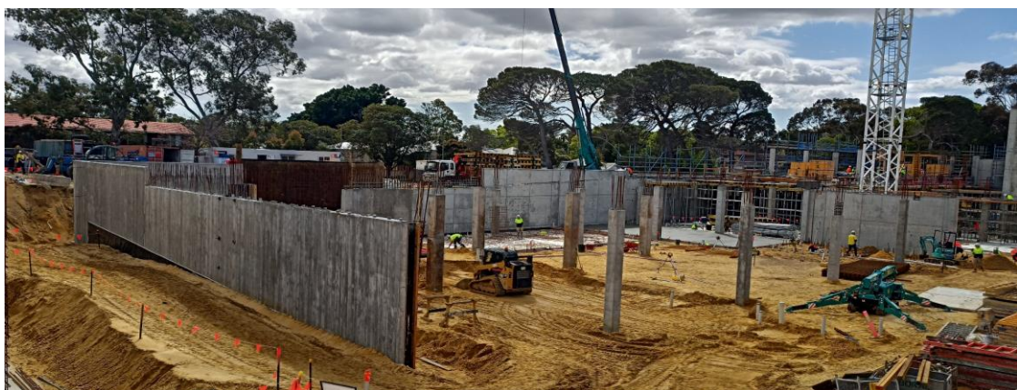
Lower ground floor looking east
