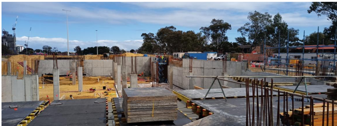
Ground floor looking west
