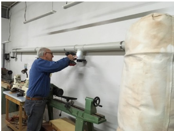
Tony Brown works on dust extraction system for wood turning area.
