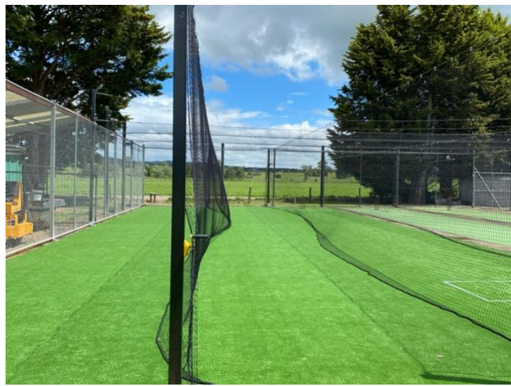
Cricket practice nets improvement project
